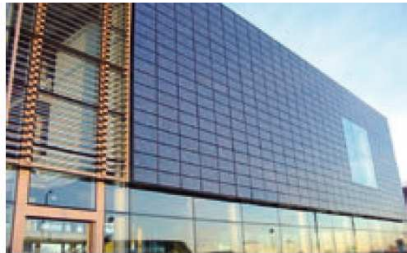
PV cladding is part of the new Manchester College of Arts and Technology (MANCAT) building, UK
