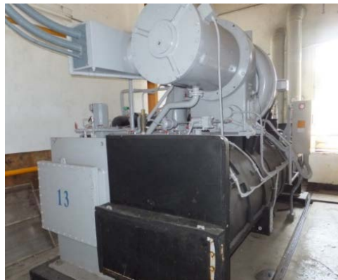
Left: High-efficiency Centrifugal Chiller, Middle and Right : High Efficiency Refrigerator
