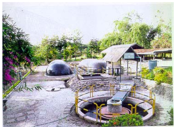
Circulation tank and biogas domes at pig farm (Pak Tho District, Thailand)
