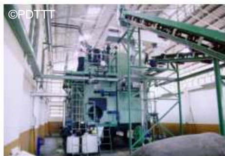
Fluidized bed boiler superheated steam, Thailand
