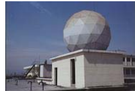
Beijing Receiving Station
