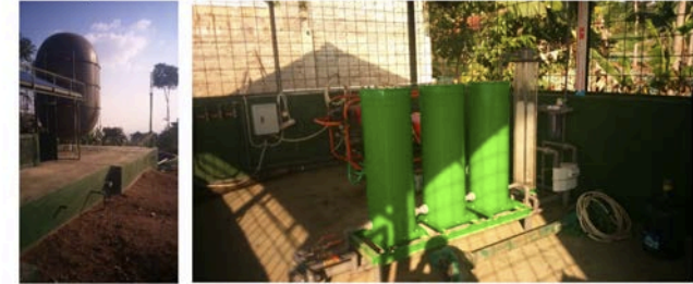
Installation of gas reactor to produce electricity for household needs
