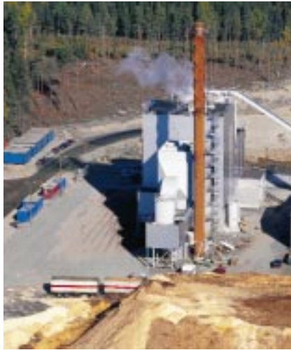
Combined production of electricity and heat from wood and waste fuels in the Forssa biomass power plant.
