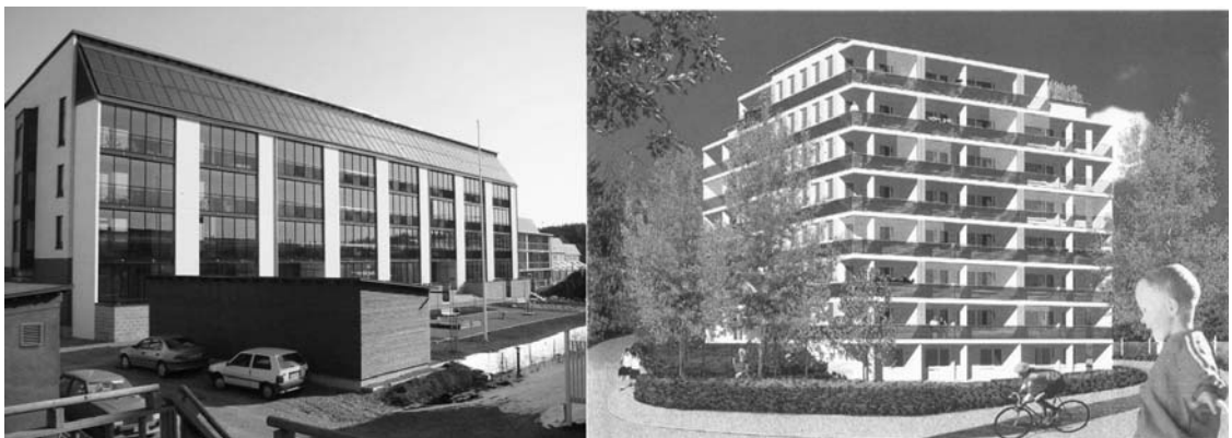
Figure 4. Left: One of the solar heating systems (solar roof) in Ekoviikki. Right: PV balcony in Ekoviikki.
